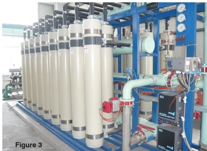
Figure 3: Vertical installation of 50m 2 elements
